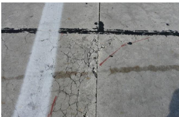
Heavily stressed concrete and asphalt pavements
