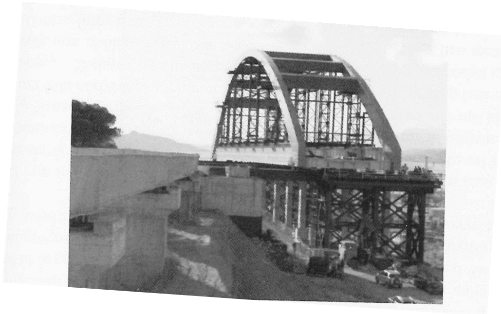
Bridge with railway line over the Ikonion landslide, during construction phase
