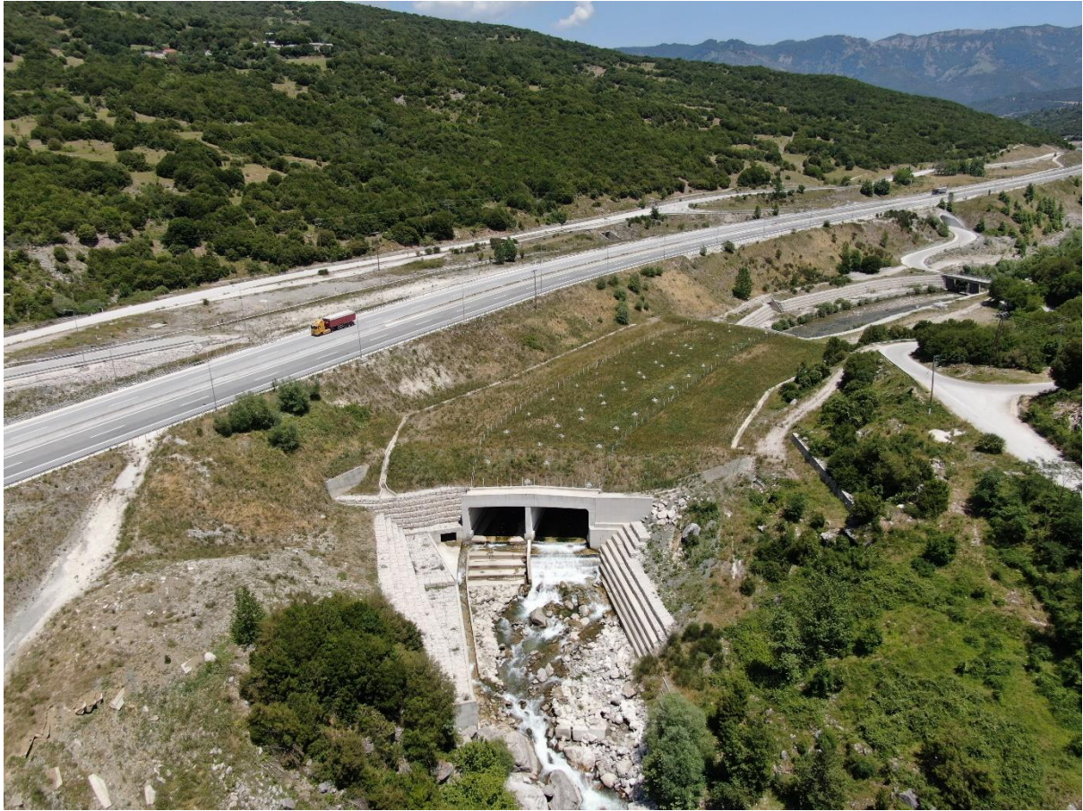
Twin tunnel of Metsovitikos River with berm above it stabilizing one landslide to the north (left side) and to the south (right side). Picture taken by drone from downstream of the river.
