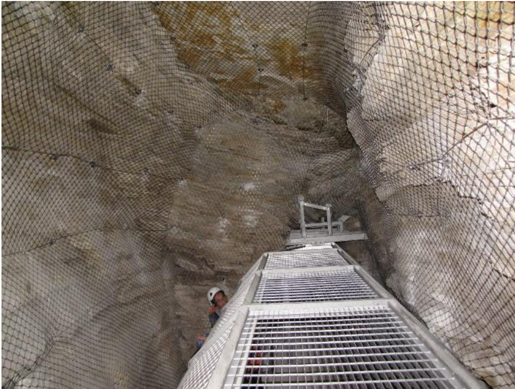
Support measures of Eupalinos aqueduct
