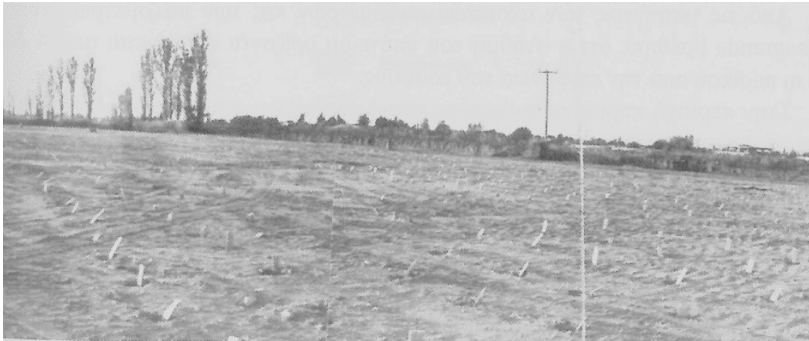
Soil improvement. Preloading with drains for the Indoor Thermi Stadium.
