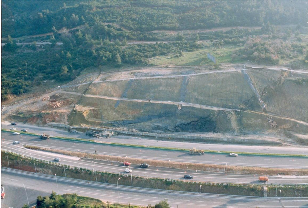
View of Malakassa landslide
