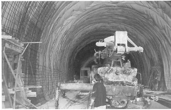
Tempi tunnel during excavation phase
