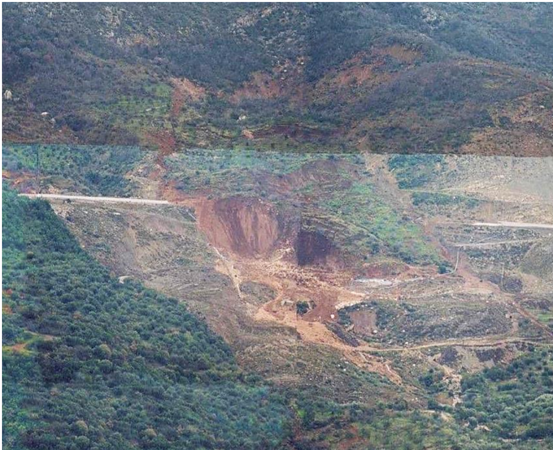
View of Tsakona landslide
