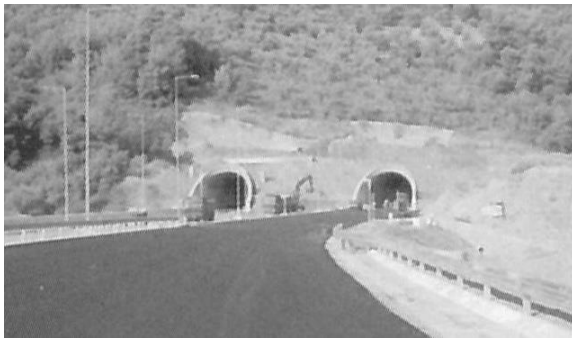
Twin tunnels of Ag. Konstantinos
