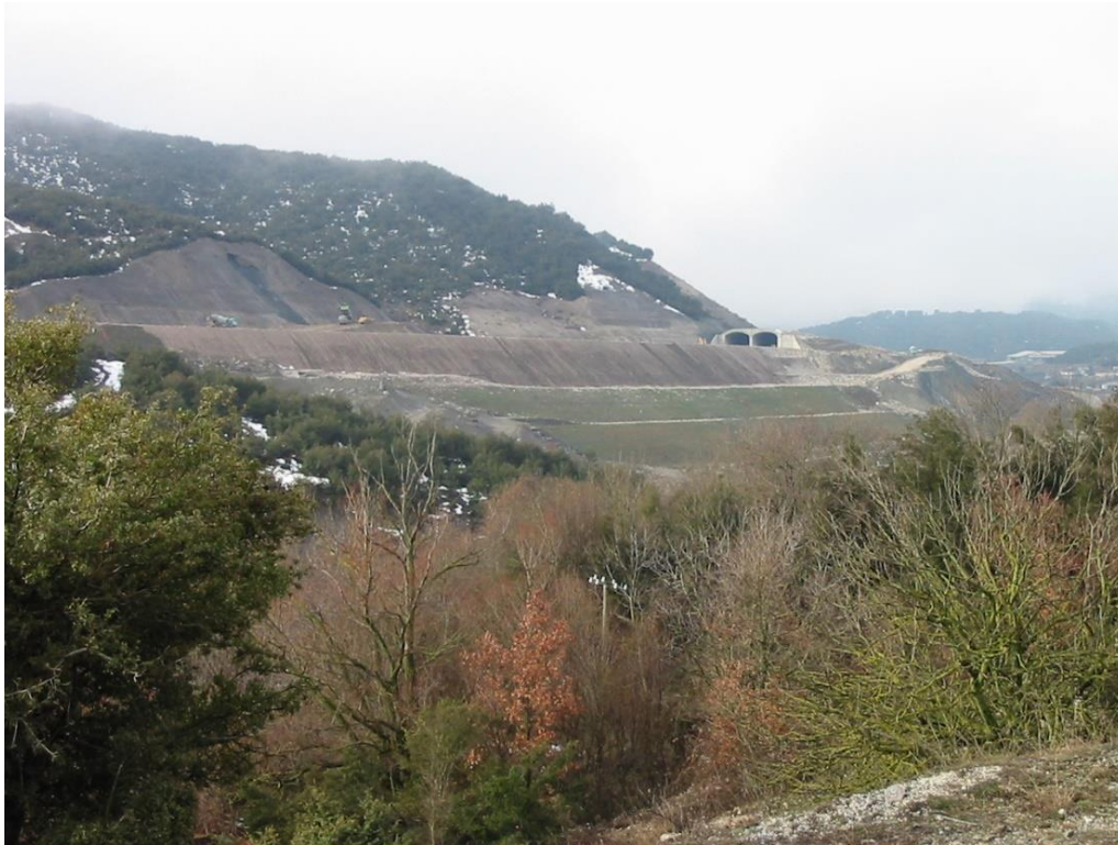
Reinforced earthfill of Egnatia Highway in Metsovo area
