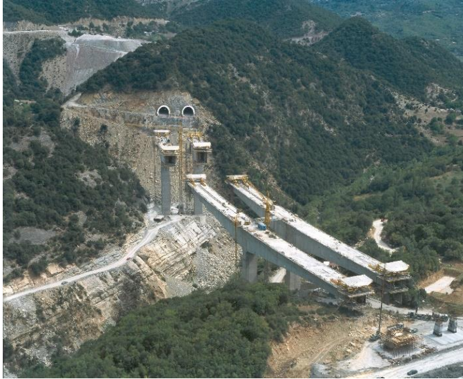
Votonossi bridge during construction phase
