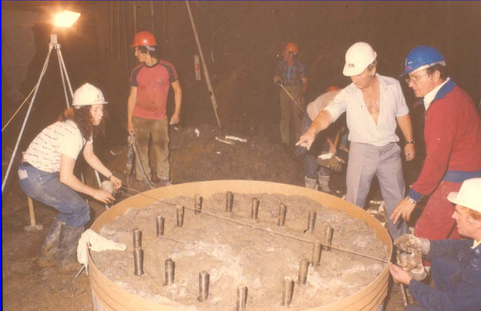
Top of pile reinforcement - threaded
