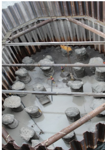
Picture 5. Sheet pile chamber, piles and under water concrete floor (Samstag & Stremmel, 2016)
