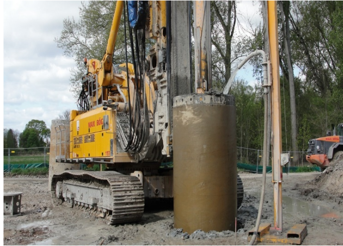
Picture 4. Diameter of piles: 1.80 m, Length: 30 m (Samstag & Stremmel, 2016)
