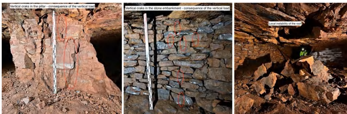
Figure 6. Example of photos accessible from the model and allowing visualization of disorders such as cracks in pillars (left) or in embankments (center) and roof instabilities (right)
