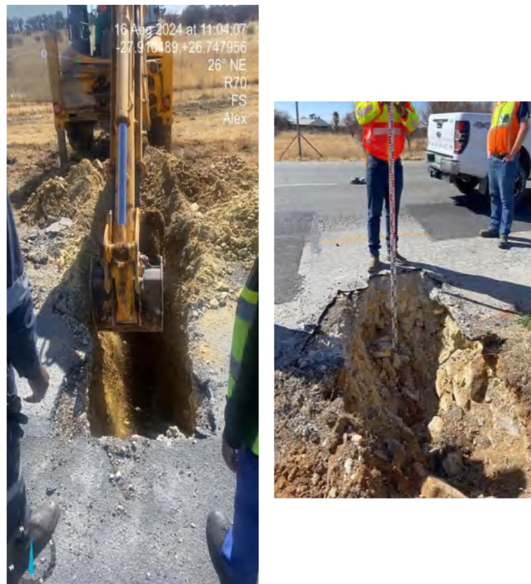
Figure 1. Excavation of testpit 1 (left) and testpit 2 (right)
