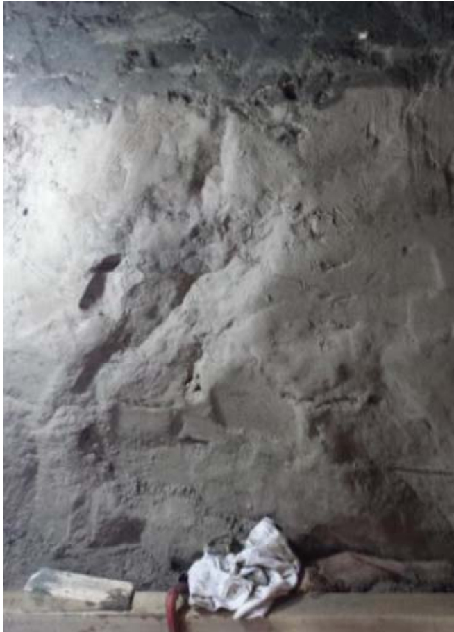
Figure 10. Photograph of TS in excavation for Cross Passage 13 (point D in Figure 1). The upper TS stood as a stable face with clear tool indentations in an open excavation, with vacuum well facilitated dewatering. Note UF-TS interface.
