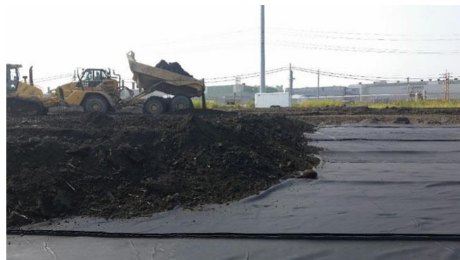
Placement of fly ash.
