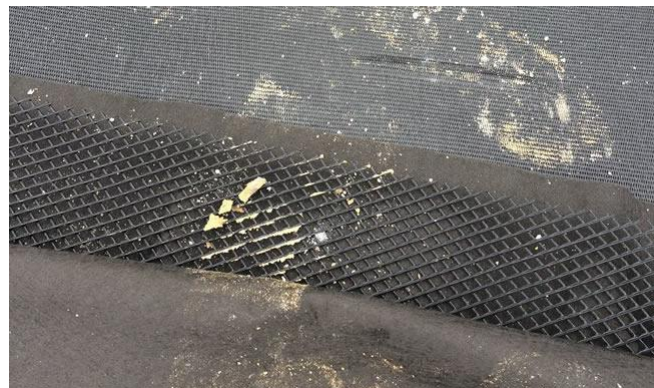
Placement of geocomposite drainage layer directly atop the geotextile
