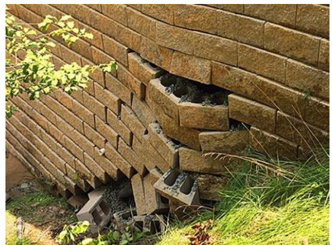
Figure 3. Toe failure of MSE wall caused by hydrostatic pressures.
