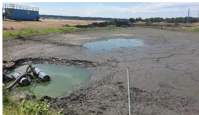
Prior to geosynthetic installation, remaining surface water from the impoundment was removed by the contractor.
