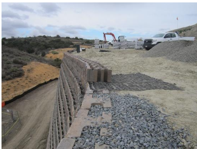
Figure 8. Secondary geogrid at wall face at Portola South project
