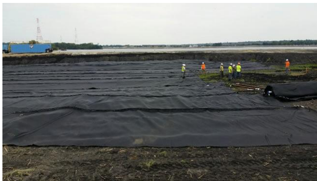
Panels were sewn in the factory into 22.9 m (75 ft) by 91.4 m (300 ft)
