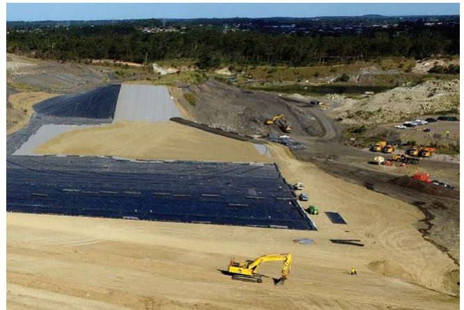
Photo of bidim geotextile installation from Geofabrics Australasia
