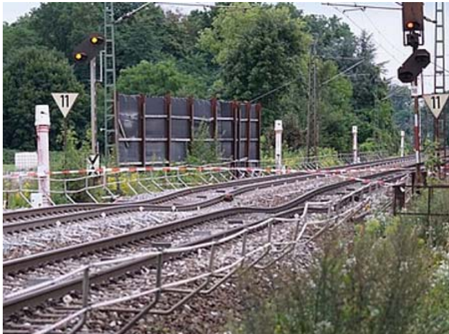
Collapse sinkhole beneath the existing surface rail tracks
