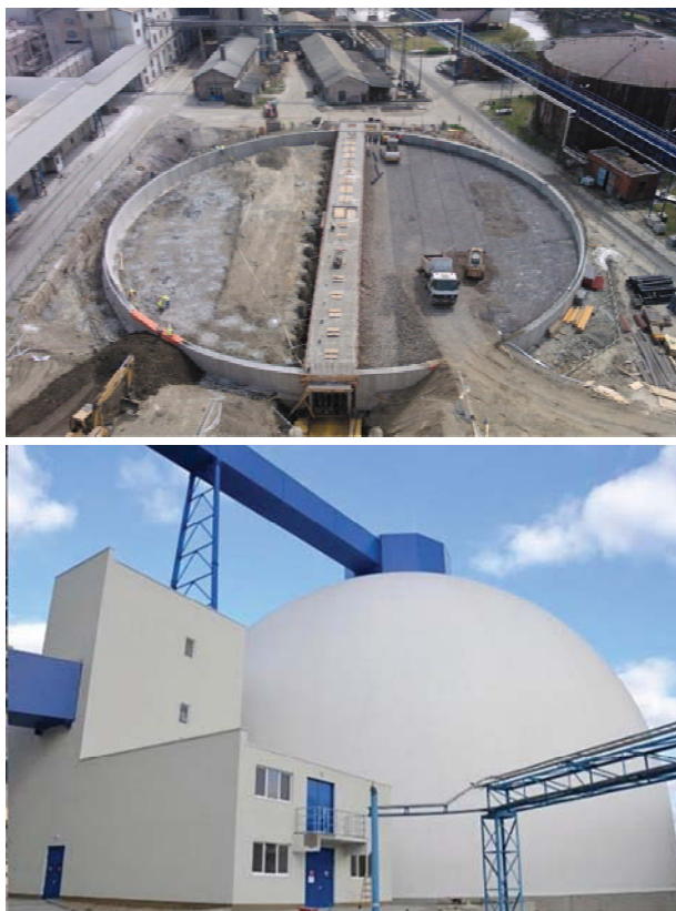
Figure 1: Pictures of the sugar silo: (a) Under construction, and (b) After completion
