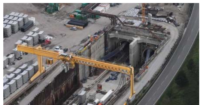
Launch and working site of the twin TBM drives
