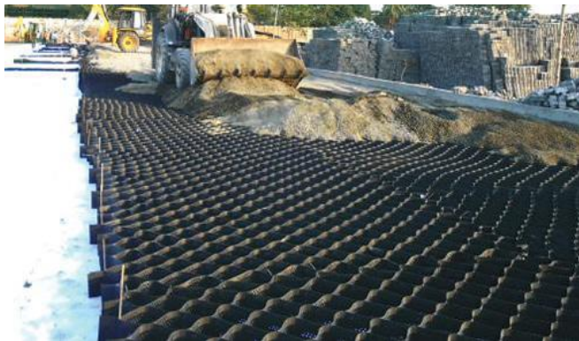
Simple placement of infill over geocell.
