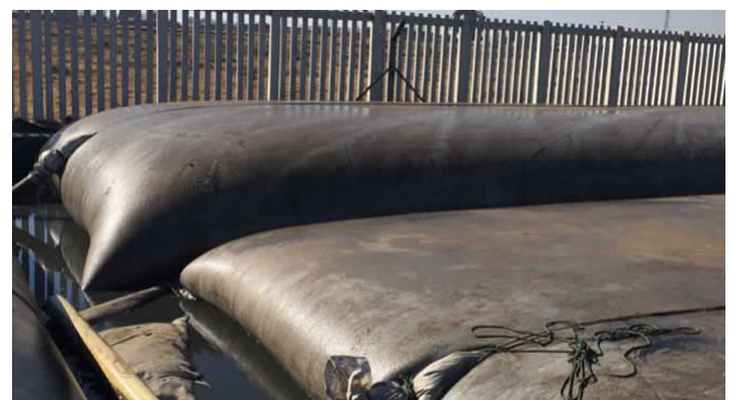
Filling of the geotextile dewatering bags.
