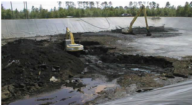
Mechanical dredging method of excess sludge from a wastewater tailings facility.
