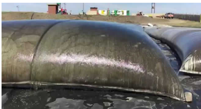
Filtration through the geotextile dewatering bags.
