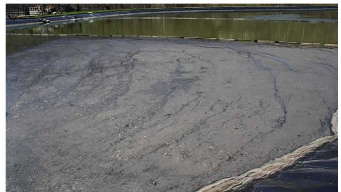
Sludge accumulation at a wastewater tailings facility.
