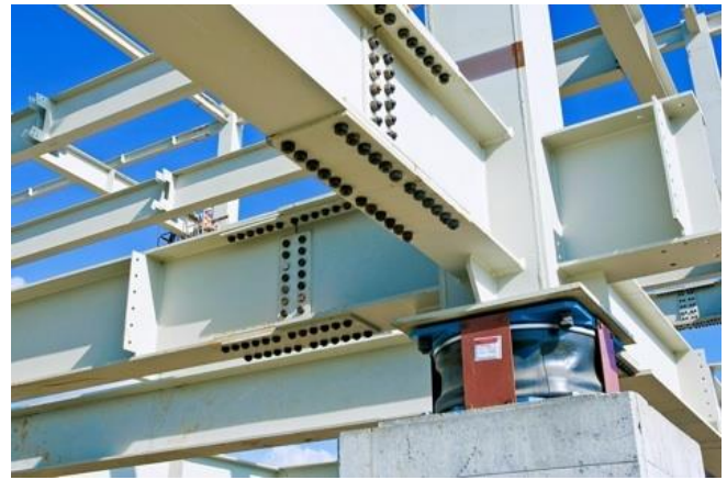
Sabiha Gökçen New International Airport, Istanbul Isolator-column-beam connection
