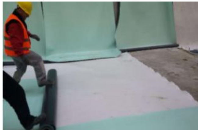
Figure 2: Geomembrane placement on top of the cushion geotextile
