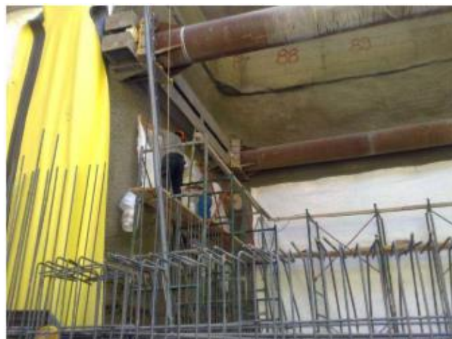
Figure 3: Cushion geotextile installation
