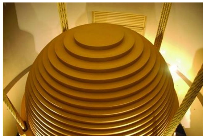
The tuned mass damper in the Taipei 101 skyscraper is a 660tonne steel sphere, made from flat circular plates welded together
