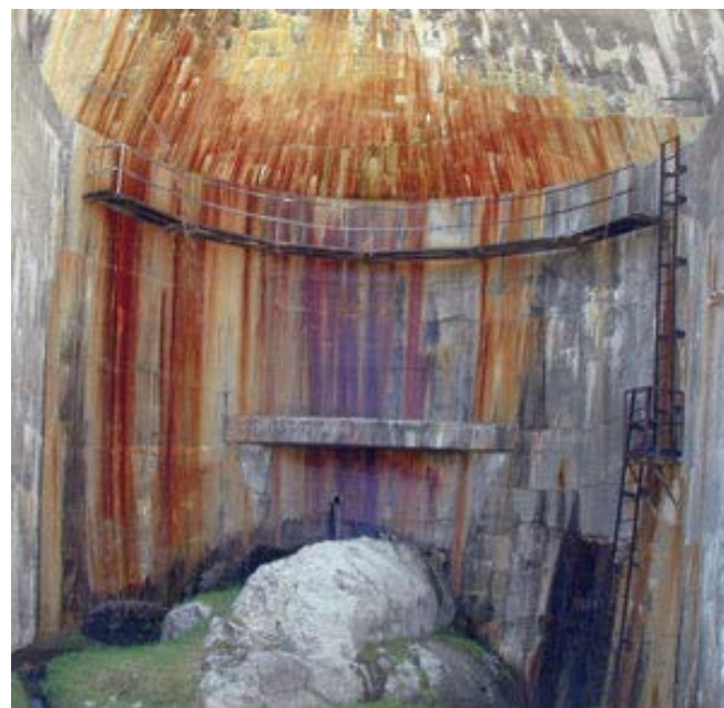
Seepage through Gem Lake Dam, completed in 1916, was severe and resulted in significant damage to the dam face.
