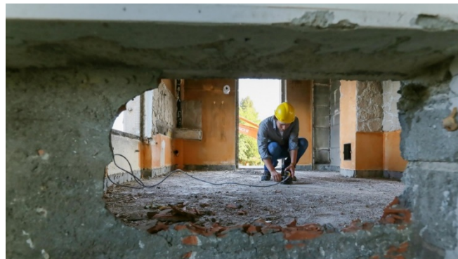
Lead researcher Yves Reuland installs a sensor in a pilot building slated for demolition.
