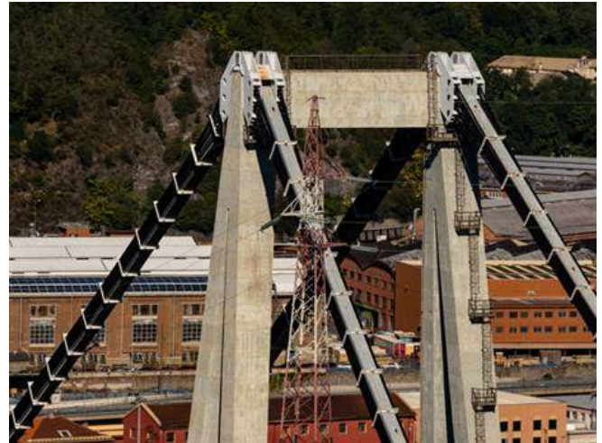
The original repairs were carried out on Tower 11 due to problems with spacing of the cables and the modifications alleviated the problem
