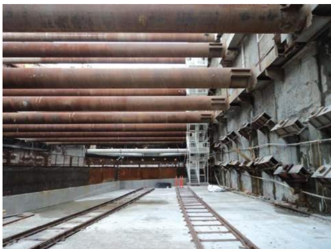
Figure 3. SOE system comprised of slurry walls, struts, and tieback anchors.
