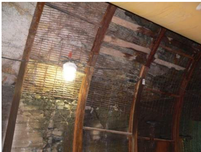
Figure 2. Shear zone in rock tunnel excavation.
