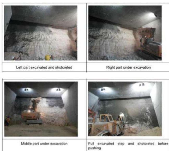
Figure 7 Excavation sequence with shotcrete application to control over-excavation
