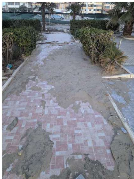
FIGURE 6. LIQUEFIED EJECTA AT THE COLLAPSED MIRAMARE HOTEL SITE.
