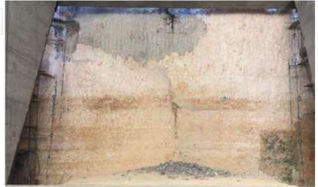
Figure 6 Example of Face Mapping on Subway 1 for good rock conditions at the face
