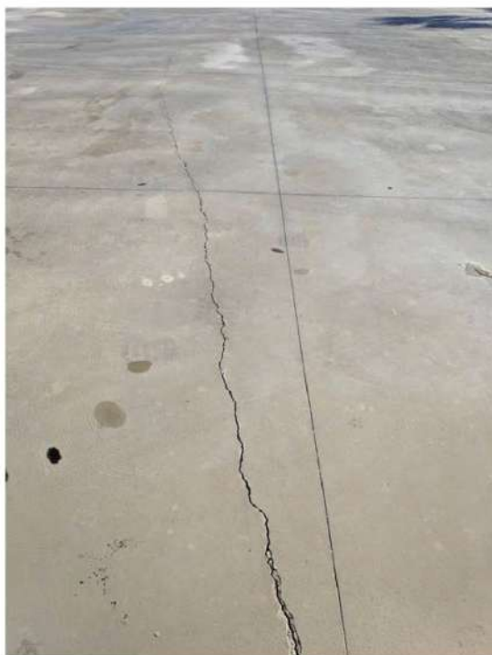
FIGURE 19. A CRACK AT A PARKING LOT NEXT TO PATOK LAGOON.
