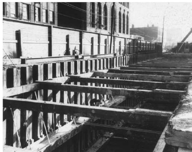
Open cut for Chicago Subway construction.
