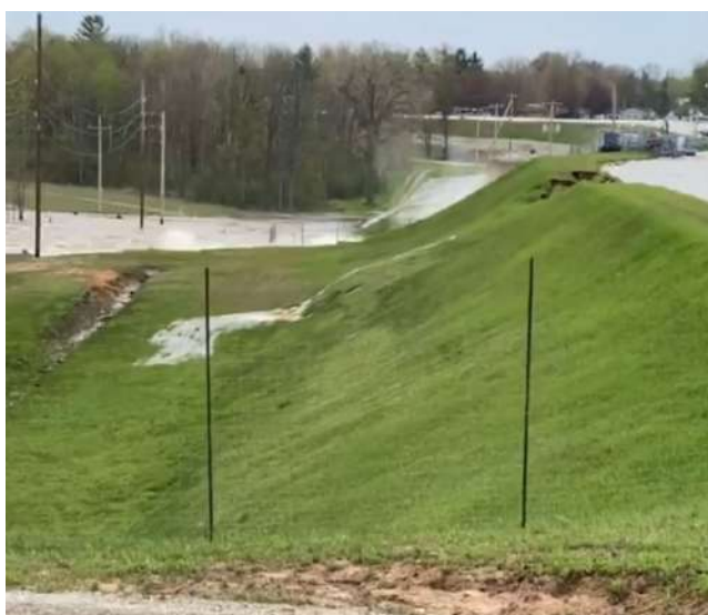
Stills from the video of the Edenville Dam failure.
