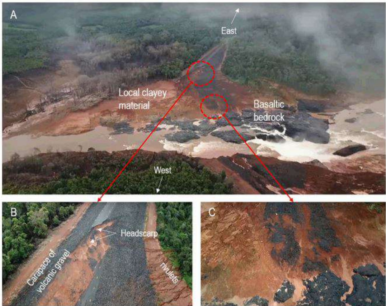
The site of the saddle dam breach at the Xe Namnoy hydropower complex in Laos. Image from Latrubesse et al. (2020) , using a drone video published at https://news.v.daum.net/v/20180803103600946?f=m .
