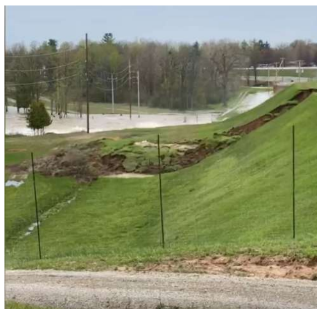
Stills from the video of the Edenville Dam failure.
