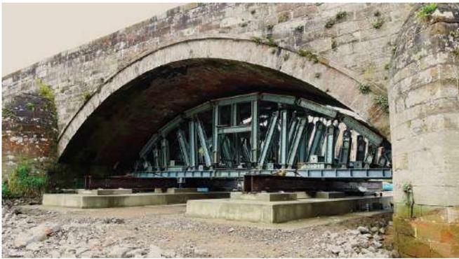
Figure 10 Centring system by temporary works specialist Mabey Contracting being rolled into position on girders on temporary spread foundations formed in the riverbed, viewed from downstream end. Note the hydraulic jacks between the tie-beam and concrete foundation bypassing the girders. The centring truss nodes each have a screw jack to fine-tune the shape up to engage the barrel intrados. Timber folding wedges are then driven into place to engage the masonry fully
