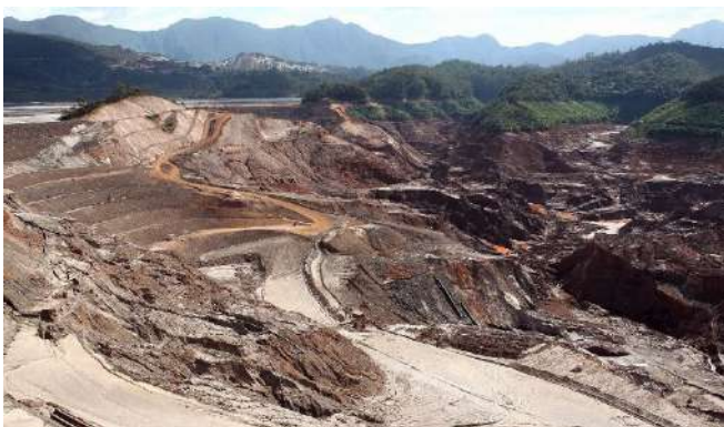
Figure 1: The Fundão Tailings Dam on the 7 July 2016, approximately eight months after failure occurred. Image courtesy of Ibama.
