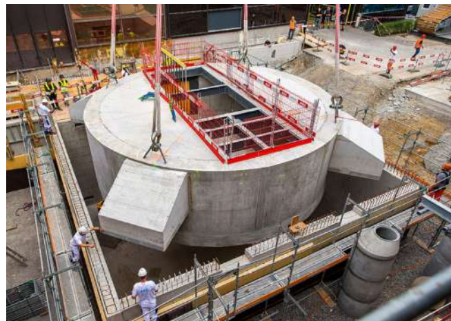
The circular concrete chamber is anchored in the ground
