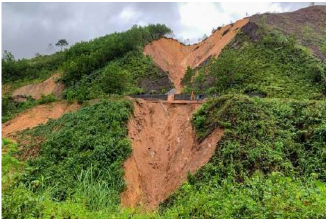
An example of landslide damage caused to a road in Vietnam
