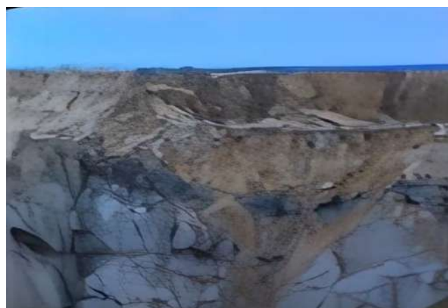
One of the rotational failures at the 1993 Pantai Remis landslide in Malaysia.
