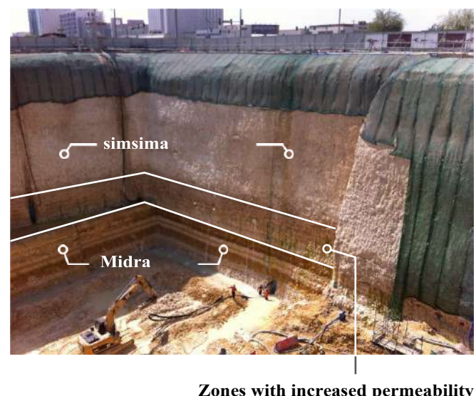
Figure 2. Zones at the interface between simsim limestone and midra shale with increased permeability, Al Matar/C-ring station of Doha metro rede line south underground.
