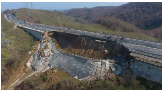
The highway slope failure at Düzce Zonguldak in Turkey on 26 March 2021
