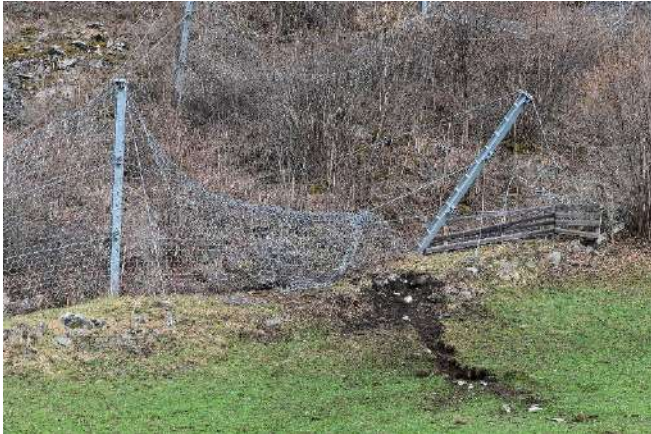
Destroyed flexible barriers along the track of the boulder that struck a house in Neustift in Austria.
