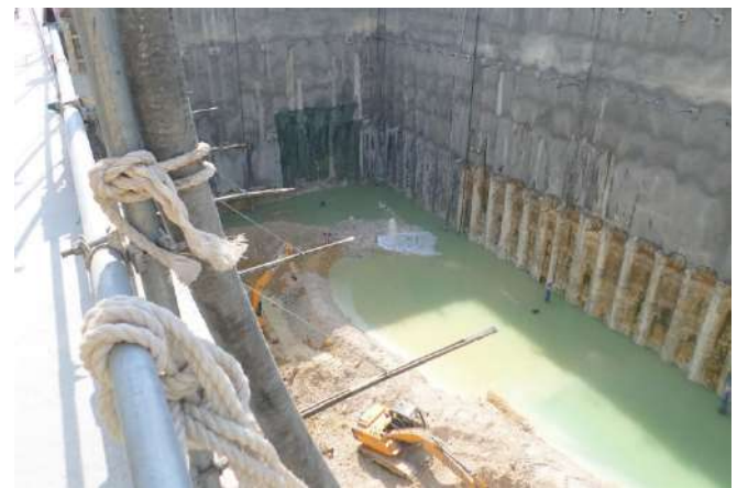
Figure 1. Flooded deep excavation after encountering a karst at Doha Souq station, Doha metro gold line underground.
