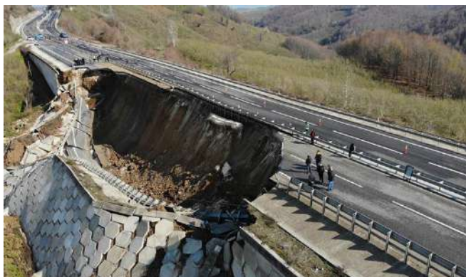
A close up view of the highway slope failure at Düzce Zonguldak in Turkey on 26 March 2021
