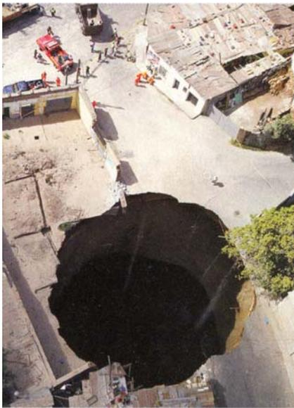
Figure 3. Leakage of a sewer pipe created a hole of 30.5 m diameter and 49 m depth in Guatemala City.
