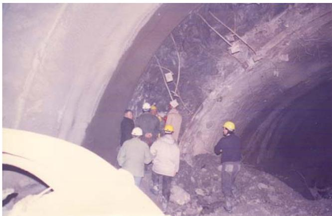
Figure 26. The maximum squeezing deformation of the Tymfristost Tunnel was as much as of 2 m.
