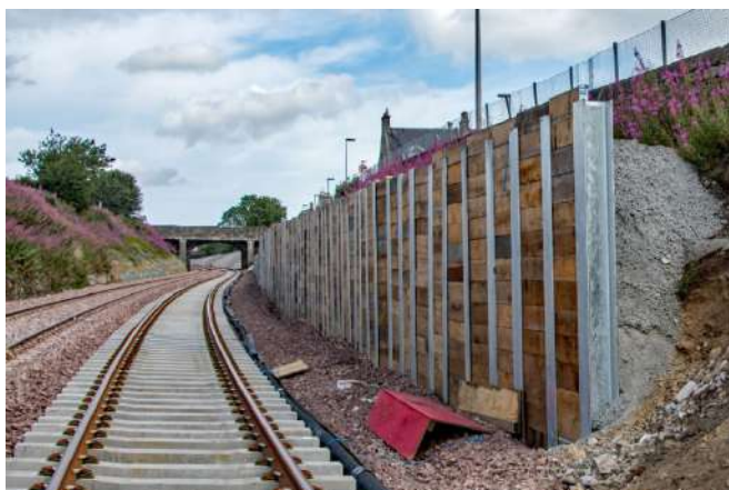
A retention wall built for double-tracking between Aberdeen and Inverurie.
