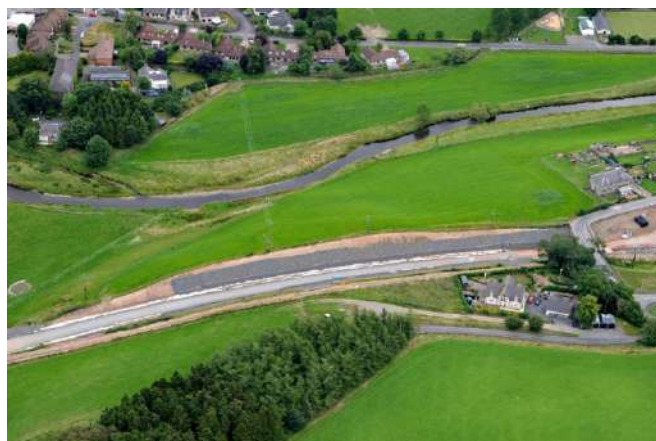
Cutting work needed to reinstate double track for the Borders Railway near Stow.
