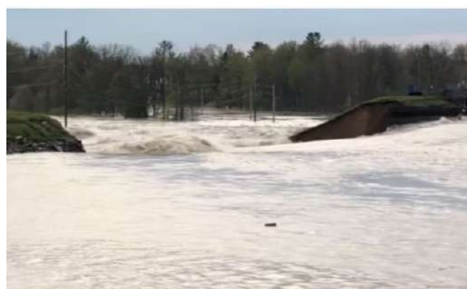
Figure 20: Edenville left embankment breach at 7:13 p.m. on Tuesday, May 19, 2020
