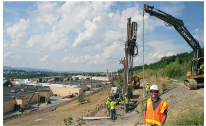
Installation of shear pins upslope from the existing failure
