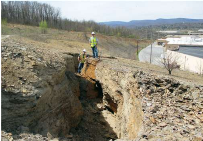
Tension crack along top of the cut
