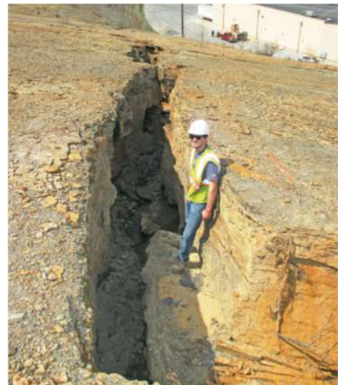
Tension crack at the back of the slide mass
