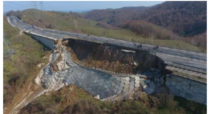
The highway slope failure at Düzce Zonguldak in Turkey on 26 March 2021. Image from Haber Gorkoy.
