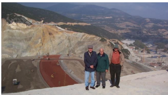
Ilarion high earthfill dam under construction in Central Greece. The Panel of Experts: Victor Milligan, Dr Evert Hoek, Prof. Paul G. Marinos (in the middle of 00's)
