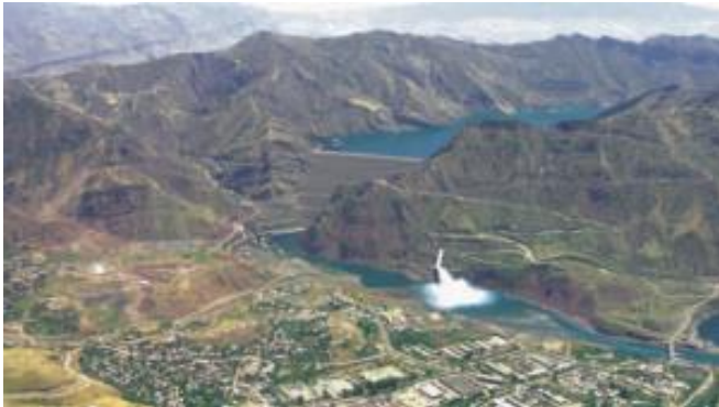
The 300m high Nurek dam on the Vakhsh river (Tajikistan)
