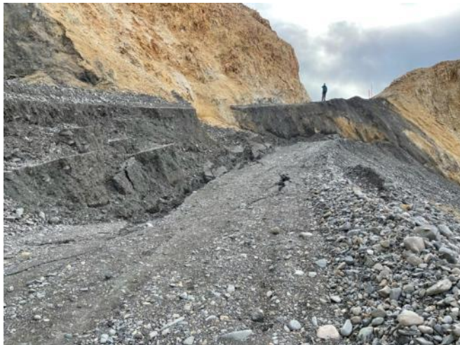
September 16, 2021 photo of eastern side of the Pretty Rocks landslide. The displacement of approximately 14 vertical feet seen below the person standing on the stable road surface (for scale) occurred over two weeks following the cessation of maintenance and road use on September 2, 2021.
