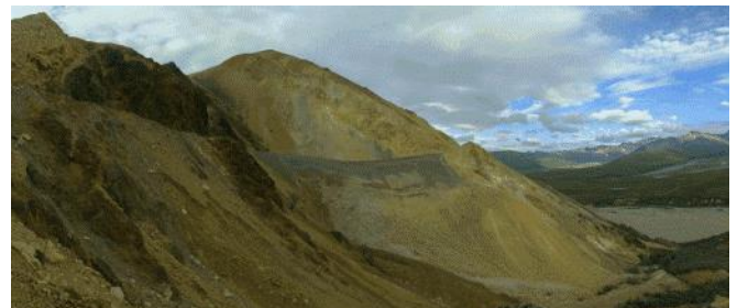
Time lapse of the Pretty Rocks slump, from July 21 to August 25, 2021. In this time, the road displacement was ~6.5 meters (21 feet)
