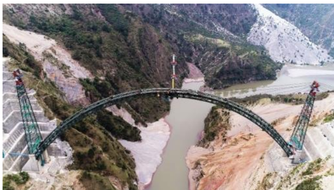
The two sides of the arch were connected in April 2021
