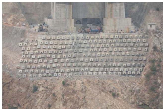
Some 237 cable anchors were installed at one of the abutting foundations (Freyssinet India)
