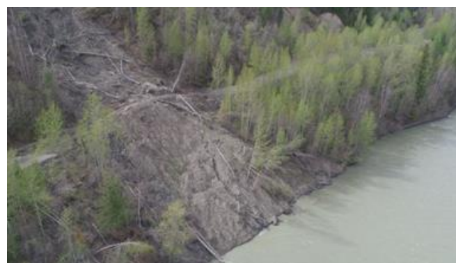
Section of Quesnel-Hydraulic Road buried by slide.
