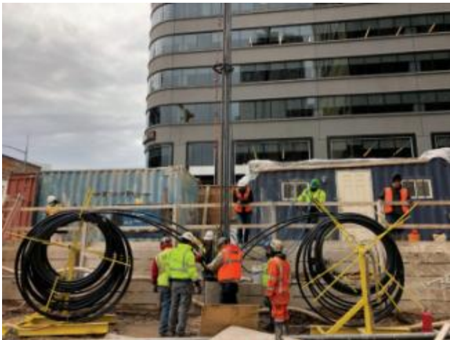
Geothermal loop installation in a pile
