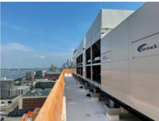
Modular rooftop heat pumps connected to energy foundations
