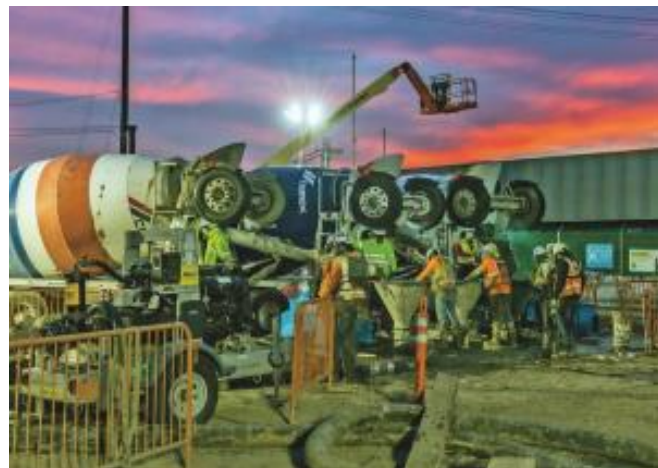
Primary panel concrete placement with simultaneous excavation in background
