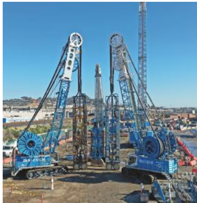
Two hydro cutters and one hydraulic grab
