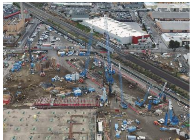
D-Wall installation
