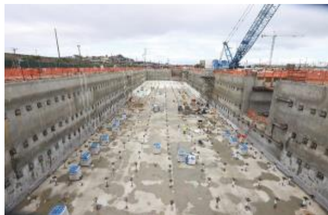
Shoring system with the excavation at full depth at Facility 610
