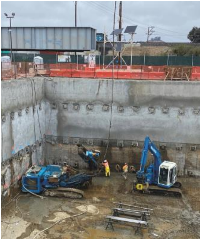
Level three tieback drilling
