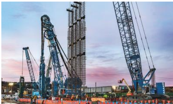
Rebar cage installation in tandem with slurry wall excavation
