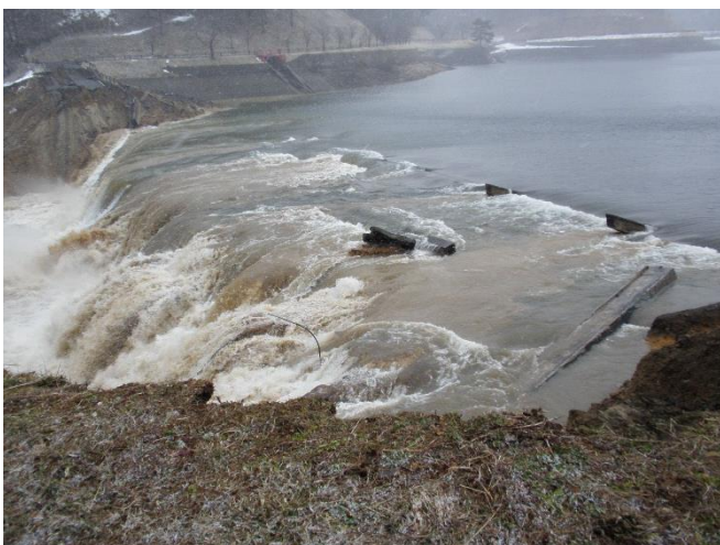
Water Overtopping Fujinuma Dam After the 2011 Tohoku Earthquake (photo by M. Yoshizawa)
