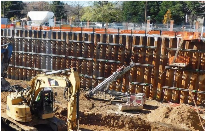
Figure 1 - Example image of steel sheet piles used as support of excavation
