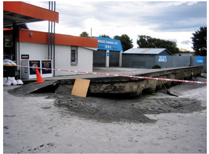
After the 2010 earthquake near Christchurch, New Zealand, liquefaction occurred throughout the city, including at this gas station. (Image courtesy of Martin Luff)
