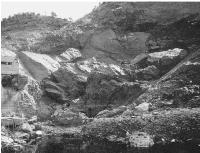
Remnants of left abutment and upstream/downstream fault lines (view from downstream) (Photo source: Richard E. Goodman, 2013 AEG Shlemon Specialty Conference).
