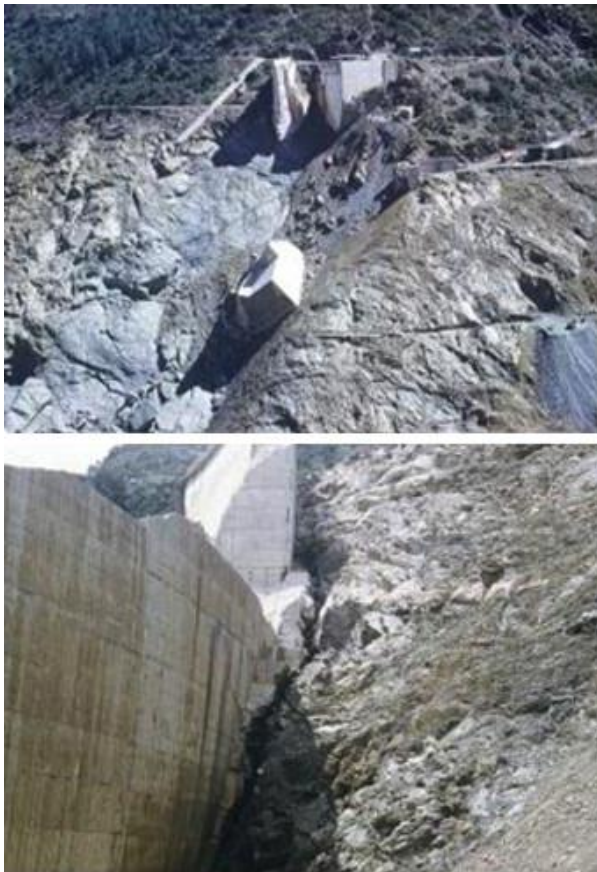
Fig. 5. The most conspicuous features of the site exposed after failure. Top, the "dihedral" excavation with half of the thrust block fallen after the flow (the exploratory adit at right was bored early after the failure to make jack tests in situ); below, a wide crevice is open just upstream of the concrete arch, wider at the base and closing more higher (photos Duffaut, 1960).
