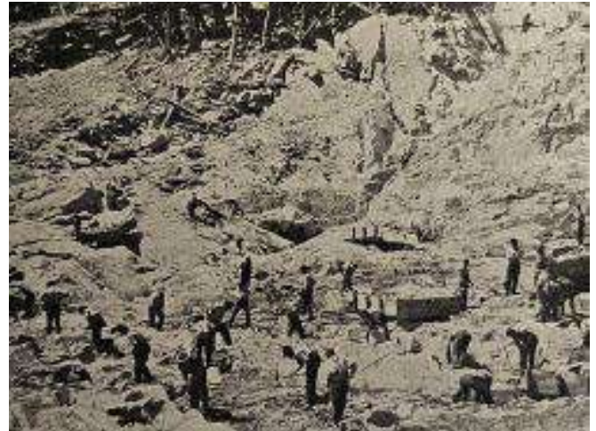
Image 15: Early stages of foundation excavation at the Arrowrock Dam, mid-1910s. Source: Baker et al. (1923).
