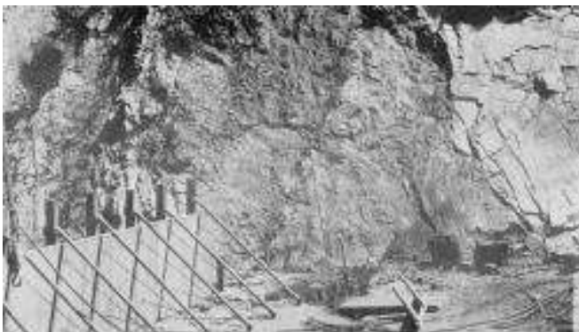
Image 21: Excavation of the east abutment of the St. Francis Dam (near location of Image 17) showing absence of a cutoff trench – a vivid departure from the Huffman Dam foundation. Source: Wiley et al. (1928).
