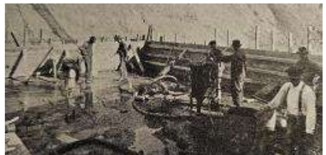
Image 19: Grouting operations for the outlet and spillway of the Lockington Dam near Piqua, OH, late 1910s. Source: Baker et al. (1923).
