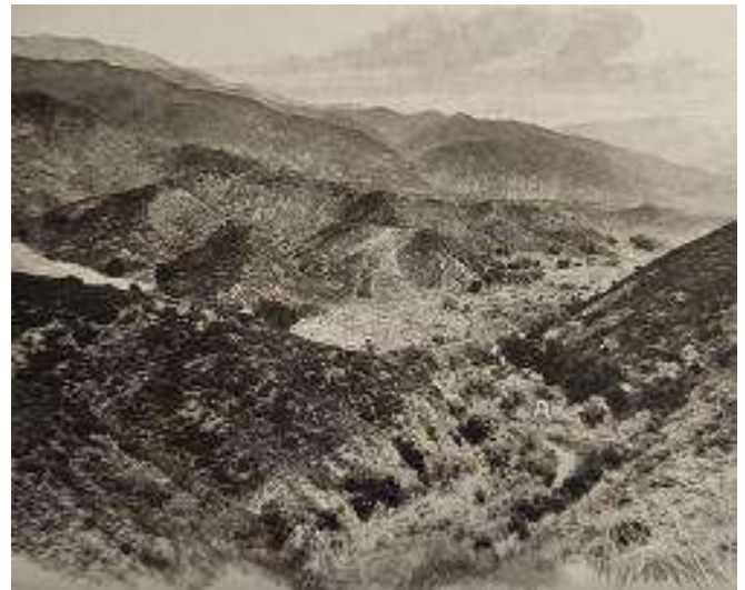
Image 13: Future site of the St. Francis Dam, early 1920s. The contact between the sandstone (dark) and mica schist (light) formations is clearly visible in the foreground; the dam's ultimate site is marked with the letter "A". Source : Hundley and Jackson (2015).
