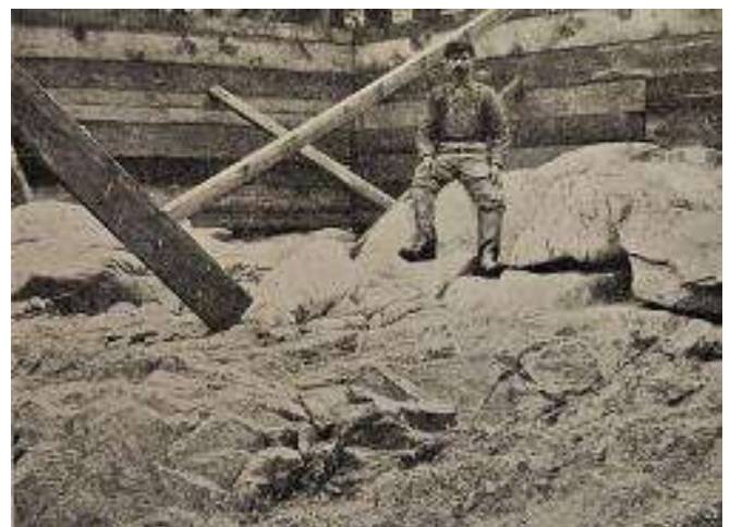
Image 16: Bedrock at the Arrowrock Dam between the completion of excavation and clean-off and concrete placement, mid-1910s. Source: Baker et al. (1923).
