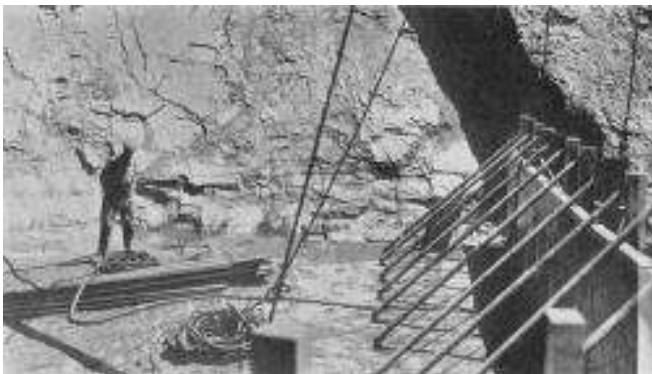
Image 17: The east abutment of the St. Francis Dam just before concrete placement, with loose mica schist clearly visible – a striking contrast with the Arrowrock Dam work. Source: Wiley et al. (1928).
