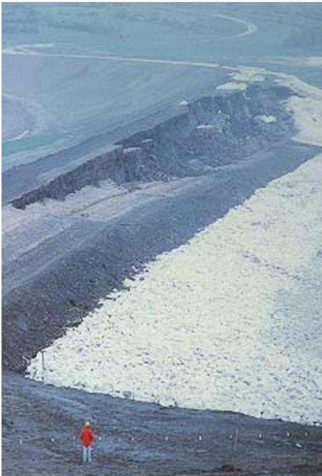
Image 7: Aftermath of the slope failure at the original Carsington Dam.
