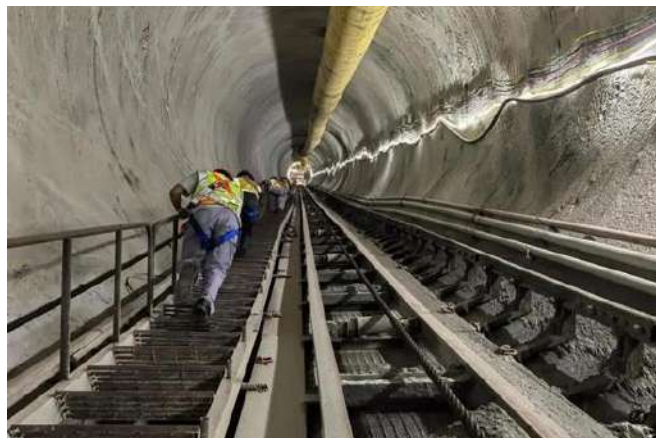
The 50 degree slope tunnelled by the TBM Tianyu
