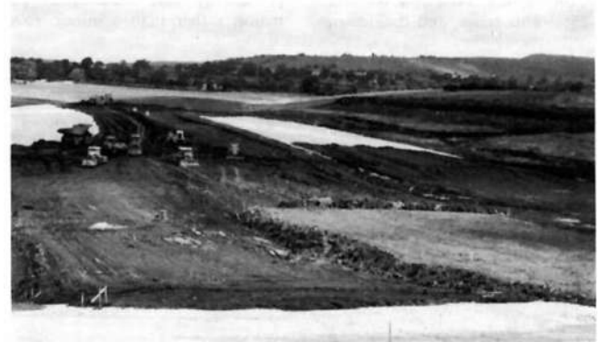
Image 5: Embankment construction progresses at the original Carsington Dam. Source: Rowe (1991).
