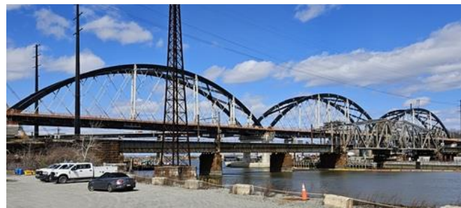
Image 25: The 1907 Portal Bridge and its replacement, April 2025. Source: Author.
