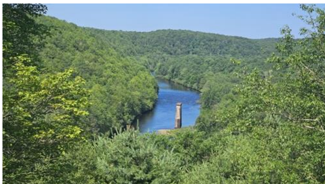
Image 23: A bridge pier from a long-abandoned branch of the Lehigh Valley Railroad stands guard in the Lehigh River near White Haven, PA. Source: Author.
