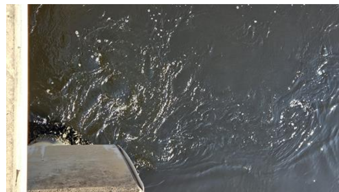
Image 22: Wake vortices downstream of the bents of a bridge over Roberts Bay in Venice, FL. The right-of-way, a former route for the Seaboard Air Line Railroad, now carries the Legacy Trail, a bicycle and pedestrian path. Source: Author.
