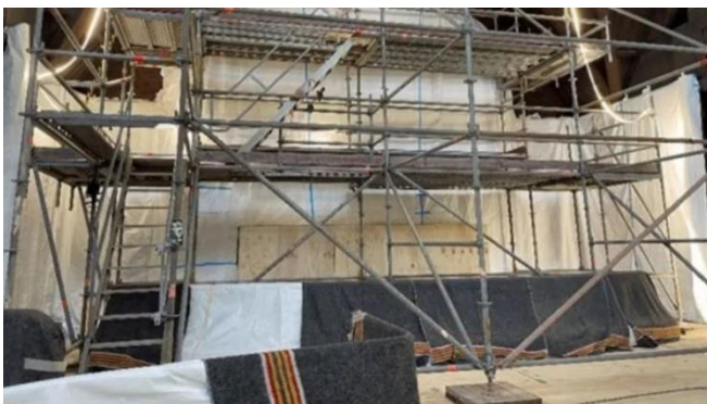
LKAB Interior parts of the church have been secured by metal scaffolding
