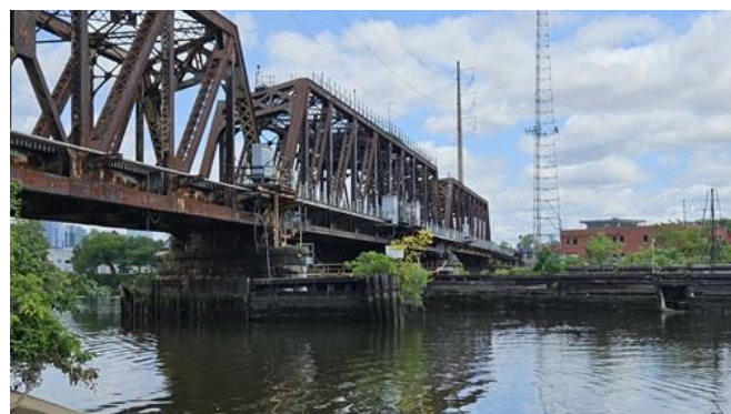
Image 26: A Lang-era B&O bridge at Bartram's Garden in Philadelphia, PA remains in daily freight use, as does the tunnel in Image 1. Source: Author.
