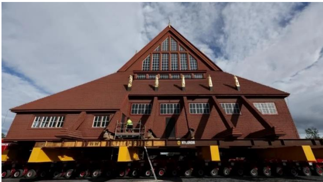
Reuters The church has been hoisted on a wheeled transportation unit
