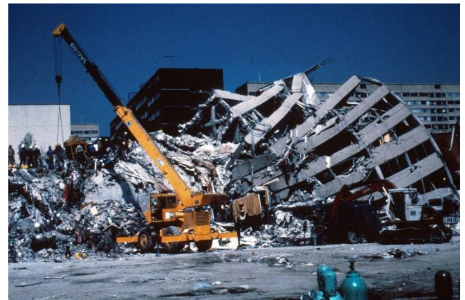
Nuevo Leon apartment building part of the structure was only slightly damaged while another part of it collapsed
