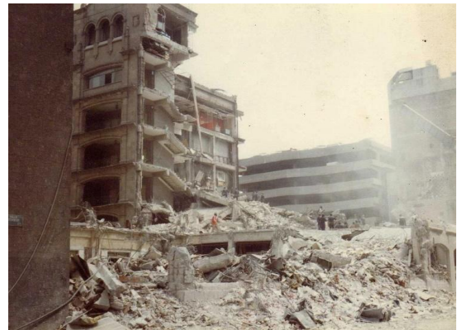
Collapsed Conalep building
