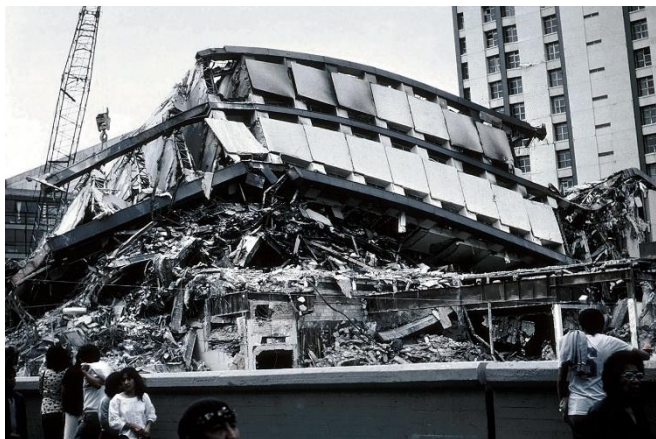
Apartment Complex Pino Suarez in the wake of the earthquake
