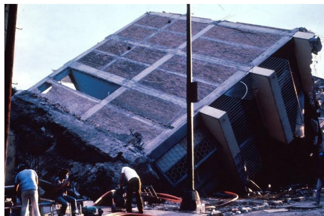
Eight story frame structure with brick infill walls broken in two. The foundation also came off
