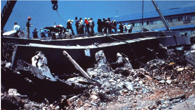
Collapsed General Hospital in Mexico City. Credit: USGS
