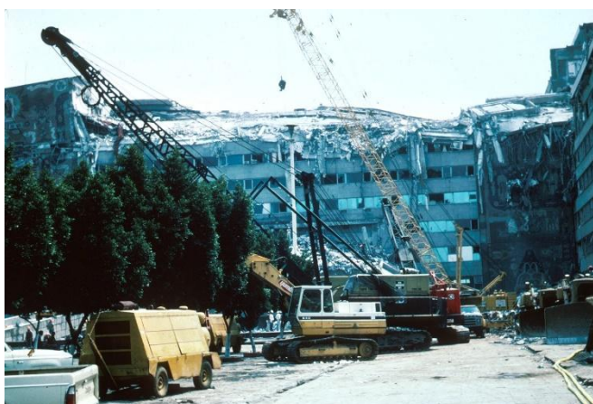
Collapsed upper stories and construction equipment at work at the Ministry of Telecommunications and Transportation building
