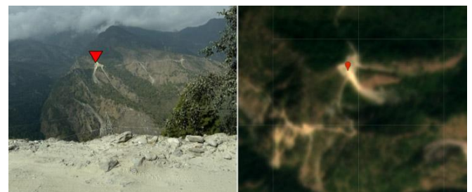
Left: A landslide near the village of Sano Haku, Nepal, indicated by the red arrow; Right: A top-down view of the landslide as seen from space (Imagery © 2025 Planet Labs).
