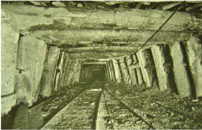
Image 10: Timbering in a subsurface anthracite mine in northeast PA, early 1900s. Source: Underground Miners (2025).
