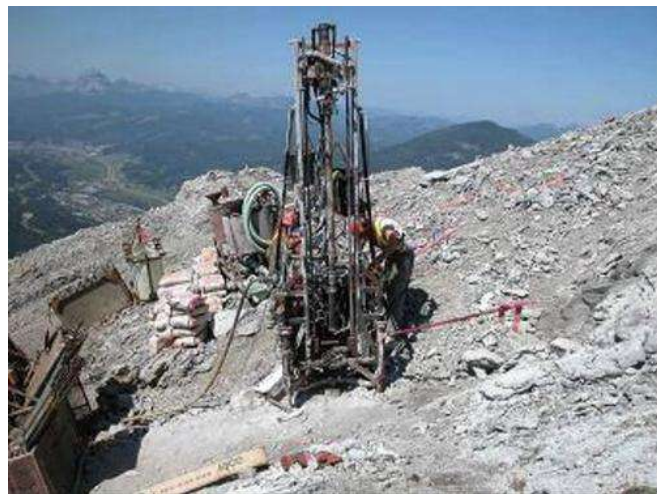
Image 25: Installation of geophones on Turtle Mountain's South Peak using a helicopter-lifted drill rig. Source: Read et al. (2005).
