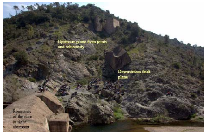
Malpasset dam failure: The students inside the dihedron removed by the uplift pressure
