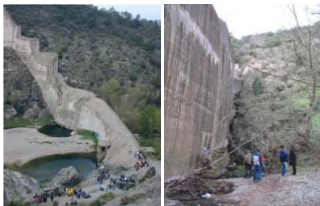
Malpasset failure: students inside the location of the uplifted wedge
