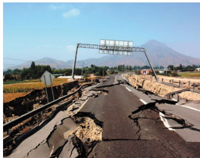
The Chile earthquake caused the liquefaction of soil under an approach to a bridge (Rob Simpson).
