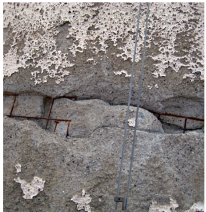
Damage to the upstream face of Gem Lake Dam as a result of continuing seepage consisted of large cracks in the gunite and deteriorated polysulfide coating.
