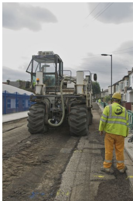
Newham Council's highways department and consulting engineer Jacobs, decided to in-situ recycle the road as it proved to be faster, cheaper and more environmentally beneficial than other options
