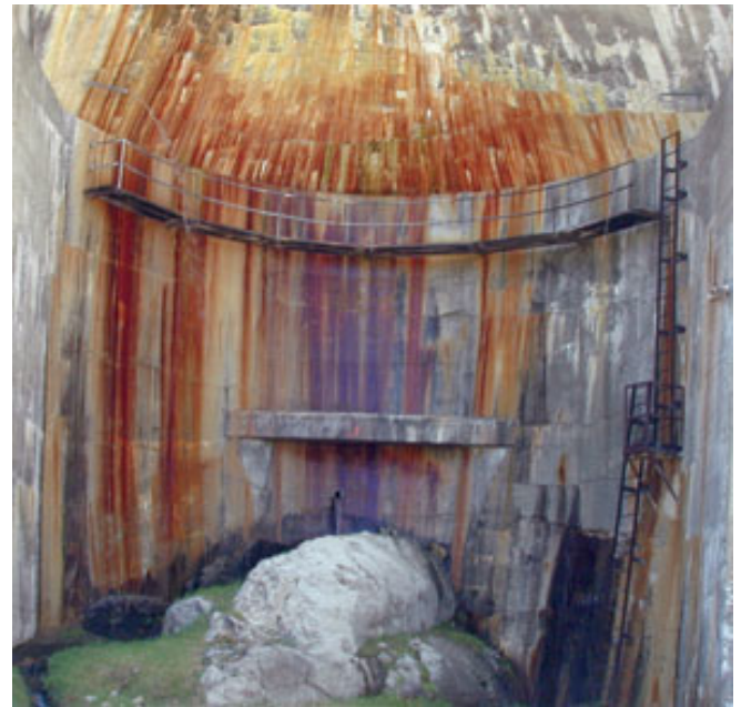
Seepage through Gem Lake Dam, completed in 1916, was severe and resulted in significant damage to the dam face.
