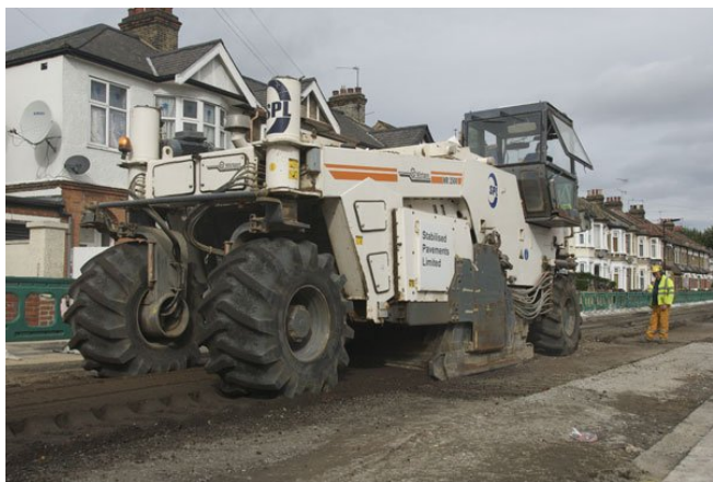
For the in-situ recycling in Newham SPL used its 500kW Wirtgen WR2500 Recycler pulverising the damaged road pavement to the required depth of 250mm
