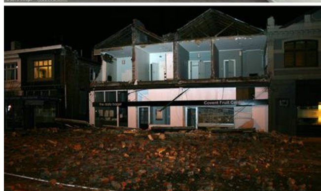
Before-and-after images of damaged buildings on Victoria Street in Christchurch.
