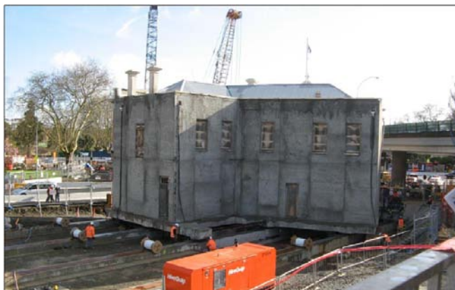
The 125-year-old Birdcage being jacked up ahead of its 40 m move to make way for the new Victoria Park Tunnel
