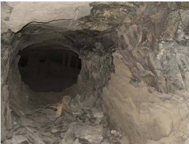
Seismic failure of a pillar holing in an intermediate-depth platinum mine
