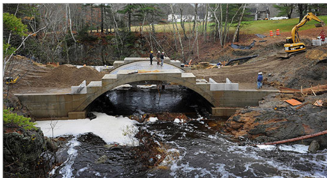
Workers construct a backpack bridge over the Little River in Belfast, Maine. (Fred Field for The Boston Globe)
