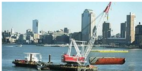
BOMBS AWAY! A crane lowers a "blanket" onto a PATH subway tunnel under the Hudson River to protect it against terrorism.
