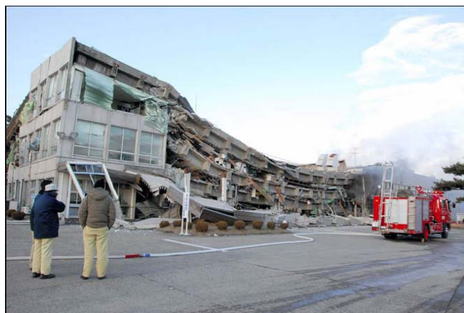
A collapsed factory building in Sukagawa
