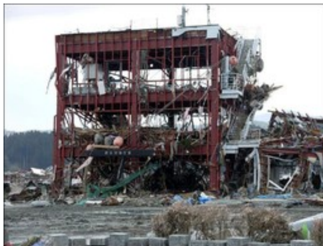
The roof of this building in Minamisanriku, Japan was a designated safe haven, but it proved insufficiently high. Around ten people managed to cling to life there, but twenty others were swept away. -- By Asian Disaster Reduction Center
