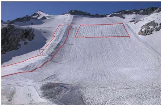
Figure 83. Local geotextile cover of glaciers to reduce melting of particular zones.
