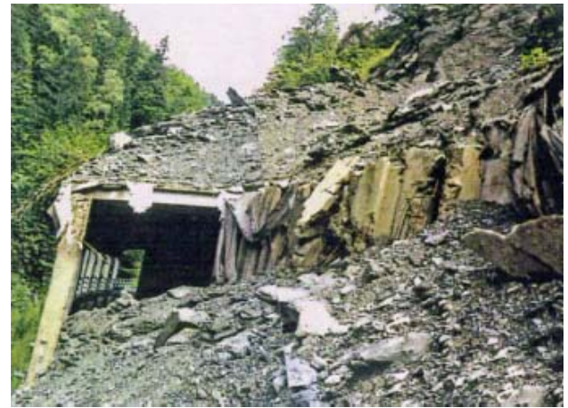
Figure 80. Damaged concrete shelter due to heavy rockfall.
