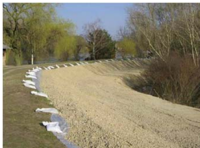
Figure 10. Hydraulic failure prevention (emergency measure) by covering the entire dam slope and berm with gravel placed on a filter geotextile.
