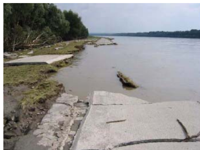
Figure 21. Stiff crest structure of a wave overtopping and spillway section of a dyke damaged by flood.
