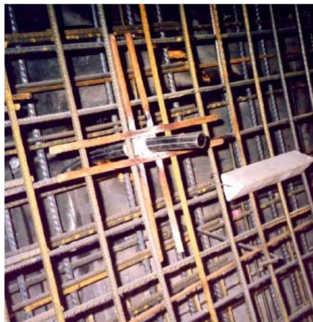
Figure 74. Pipe passage through the secondary (= inner) tunnel lining. Detail with criss-cross reinforcement.
