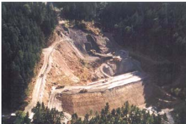
Figure 47. Rockfall barrier (geosynthetic reinforced earth dam) with upslope catch basin for 300 000 m 3 .
