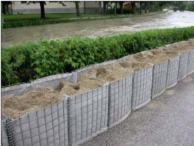
Figure 12. Mobile flood protection system with metallic gridboxes lined with non-woven geotextiles and filled with sand. Structure finally withstood a 100-year flooding event.
