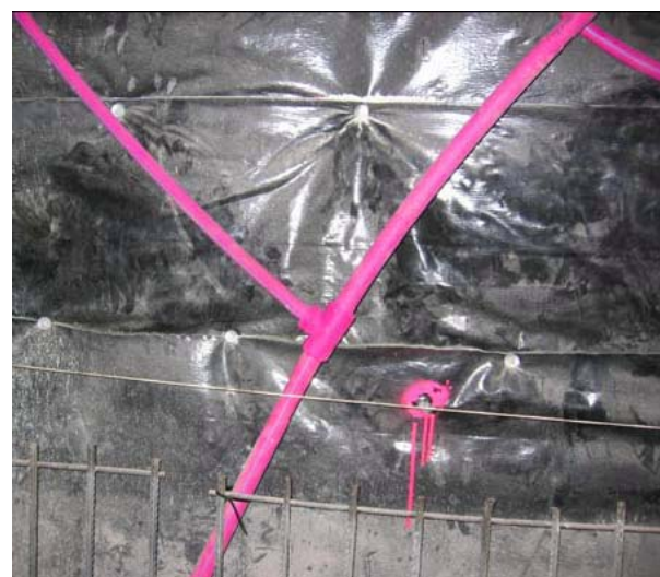
Figure 75. T-shaped elements to connect the absorber pipe from the individual strips of energy geosynthetics to the collector pipes.
