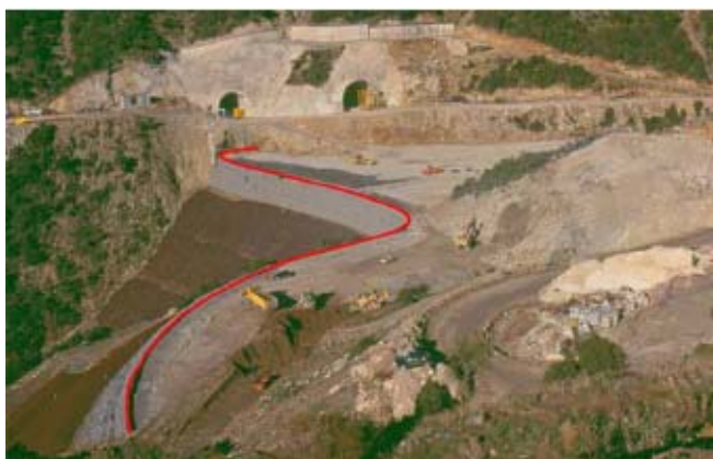
Figure 52. 60 m high geosynthetic-reinforced floating embankment in rugged steep terrain and seismic zone.
