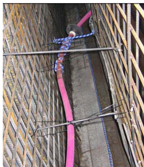
Figure 76. Collector pipe running between the inner and outer reinforcement of the tunnel lining.
