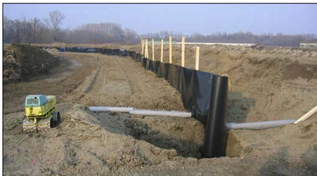
Figure 22. Back-filled geomembrane cut-off wall for low flood protective dams.
