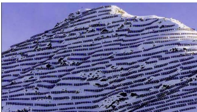
Figure 35. Protective fences to prevent the formation of avalanches already on top of a mountain.
