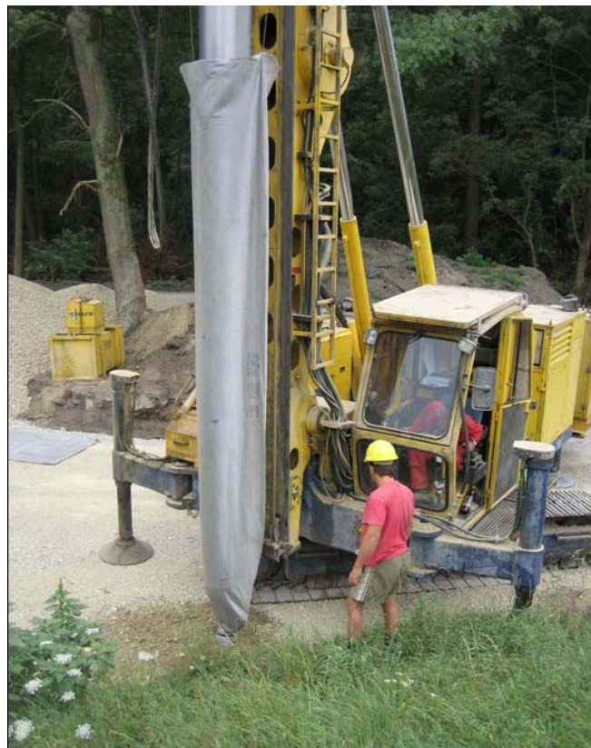
Figure 17. Installation of geotextile jacketed drainage columns (relief gravel columns) by bottom-feed vibroflotation.
