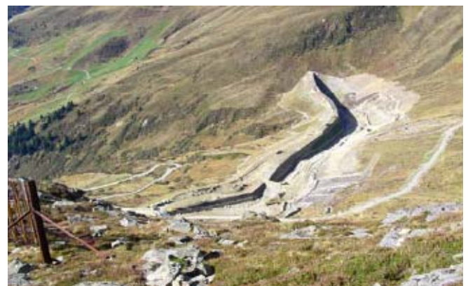
Figure 50. Barrier dam against avalanches: 500 000 m 3 L = 600 m, H = 27 m.
