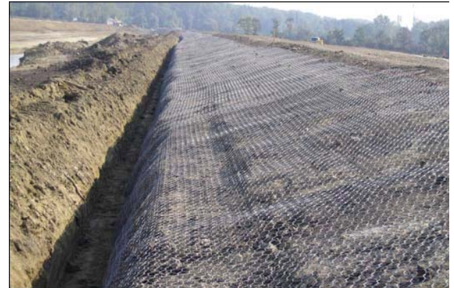
Figure 85. Installation of nets against beaver actions along flood protective dams.
