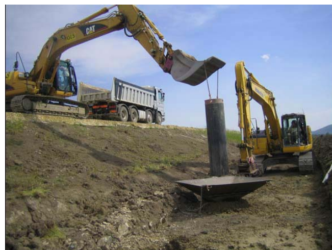
Figure 18. Installation of geotextile jacketed drainage columns by inserting a sleeved steel pipe into a pre-bored pile excavation. After pipe withdrawal, the gravel-filled geotextile hose remains in the ground.
