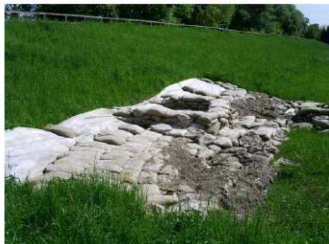
Figure 9. Hydraulic failure prevention by covering local water outflow with permeable sandbags (geotextile hand bags).
