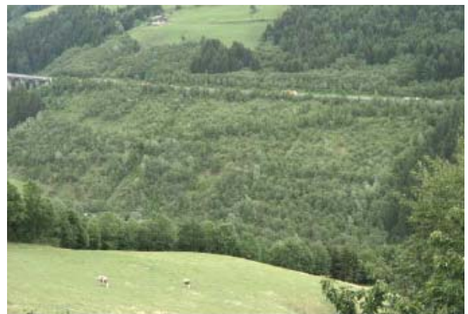
Figure 60. 120 m high embankment (large scale counterweight) instead of a highway bridge in a creeping slope, 25 years after construction.
