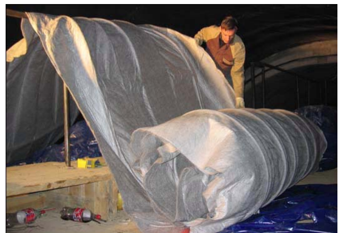
Figure 69. Unrolling of an energy geotextile (geocomposites).
