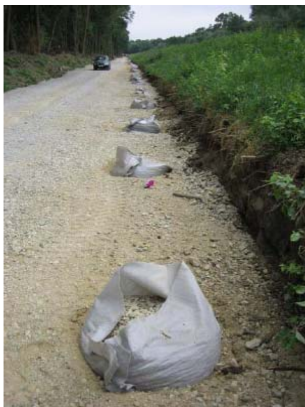
Figure 19. Top of geotextile jacketed drainage columns embedded in coarse drainage layer as sub-base of the access road for quick dam defense in case of severe floods.
