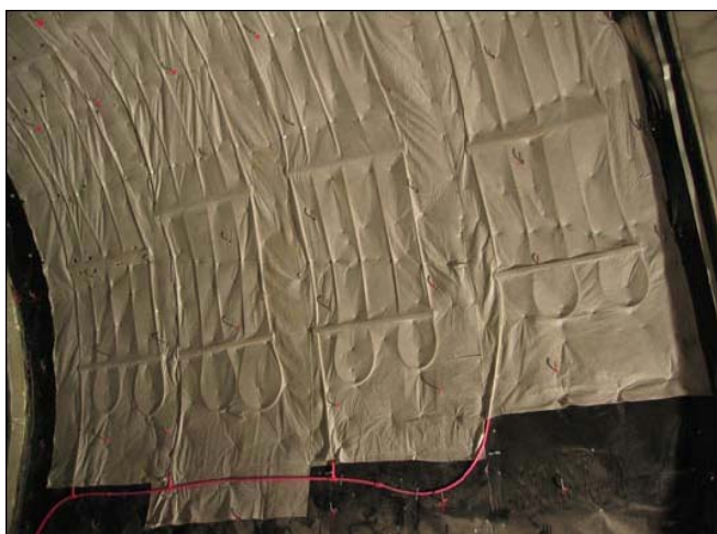
Figure 72. Installation of energy geotextiles at the testing plant „LT22 – Bierhäuselberg“. Pipe loops clearly visible.
