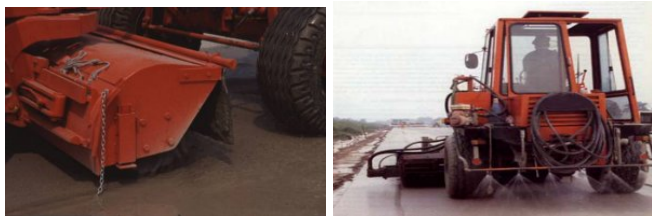
Figure 3 – Close up of brushing for surface mortar removal
