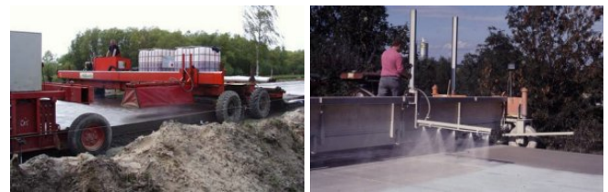
Figure 1 – Applying surface retarder and curing compound (left) or plastic film (right)
