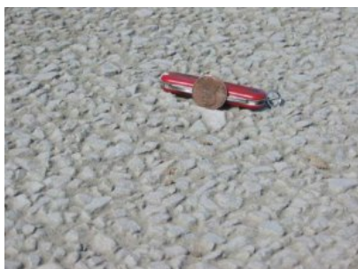
Figure 15 – As-constructed EAC surface on Kansas project
