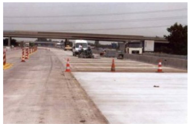
Figure 2 – Sawcutting operations followed by brushing for surface mortar removal
