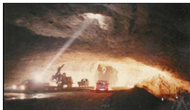
Figure 5. The UDEC-BB model shown above, gave a good (Class A) prediction of 7 to 9 mm down-ward movement. (Barton et al. , 1994). A view of the huge (stages 1 to 4) top-heading is shown.
