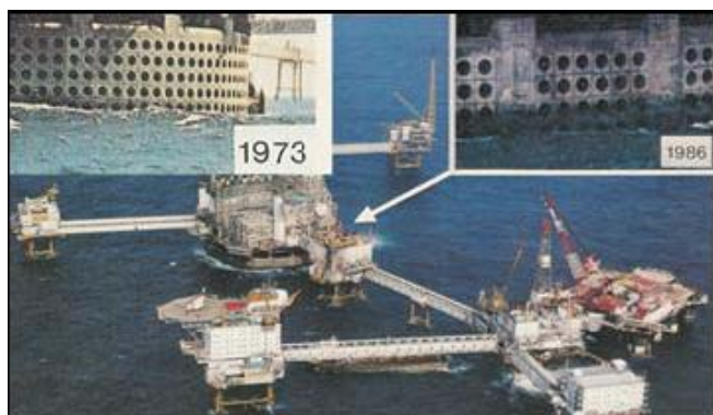
Figure 9. A view of the Ekofisk reservoir in the North Sea, where compaction of the jointed-chalk reservoir of 300 m thickness at 3 km depth caused increasing sea-bed subsidence that amounted to about 4 m when investigations began in 1985-1987. Now it is 10m.
